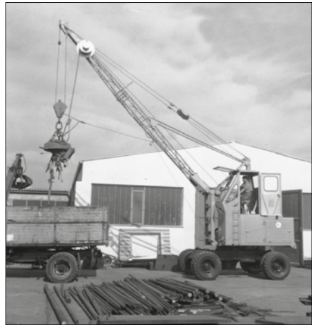
1962: rope-driven S833 with elevated operator cab
